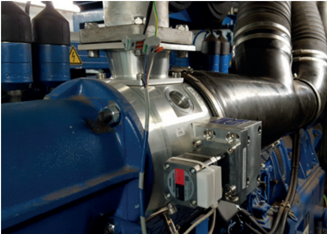
3 VariFuel2-TEM with stepper motor
